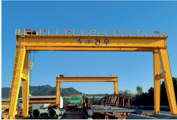
20TON GANTRY CRANE
