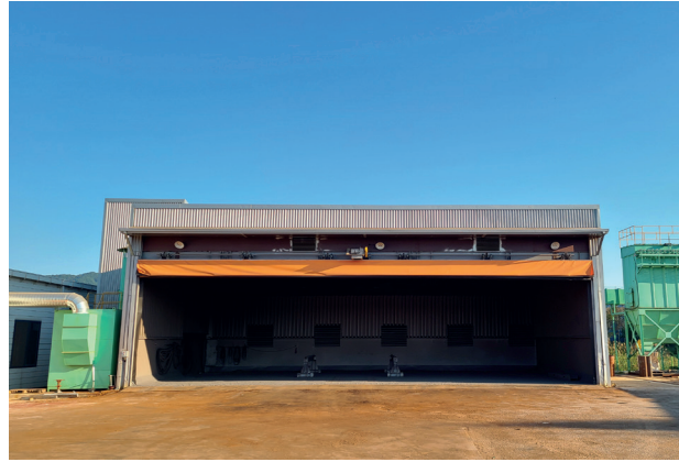
AIR BLAST SHOP
